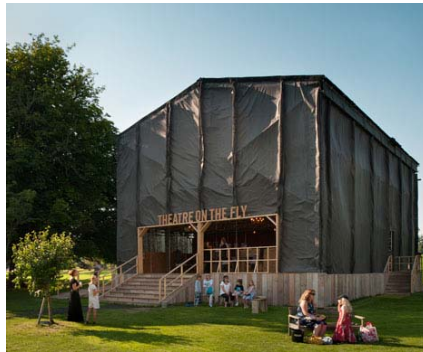
Figure 2. main facade of theater
