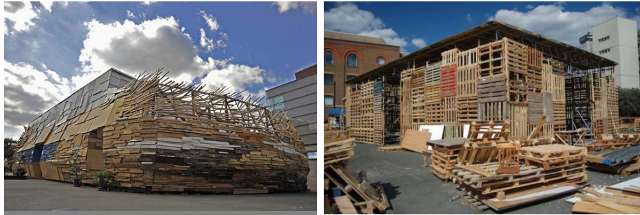
Figure 1. (a) main facade, (b) back facade
